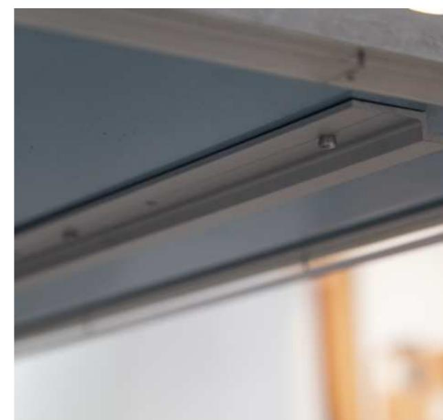
The back can be equipped with aluminium hardware to facilitate attaching the frame to the wall.
